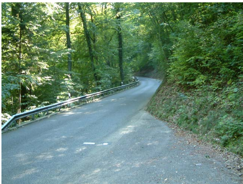
Figure 2 Photograph of the road in RV-R
